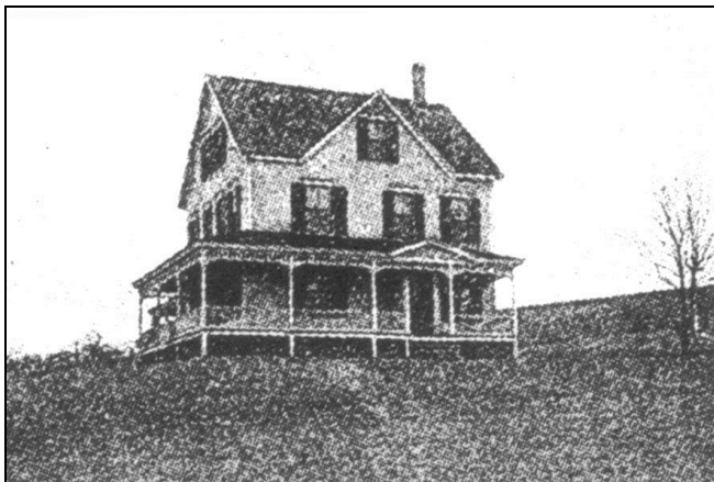
As farm house prior to conversion in 1912
