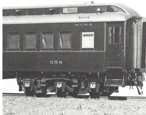
A *New York Central* coach, 1921, showing vertical end-frame flexible connector for enclosed vestibule, from John H. White, Jr., Vol. 1, p.156
